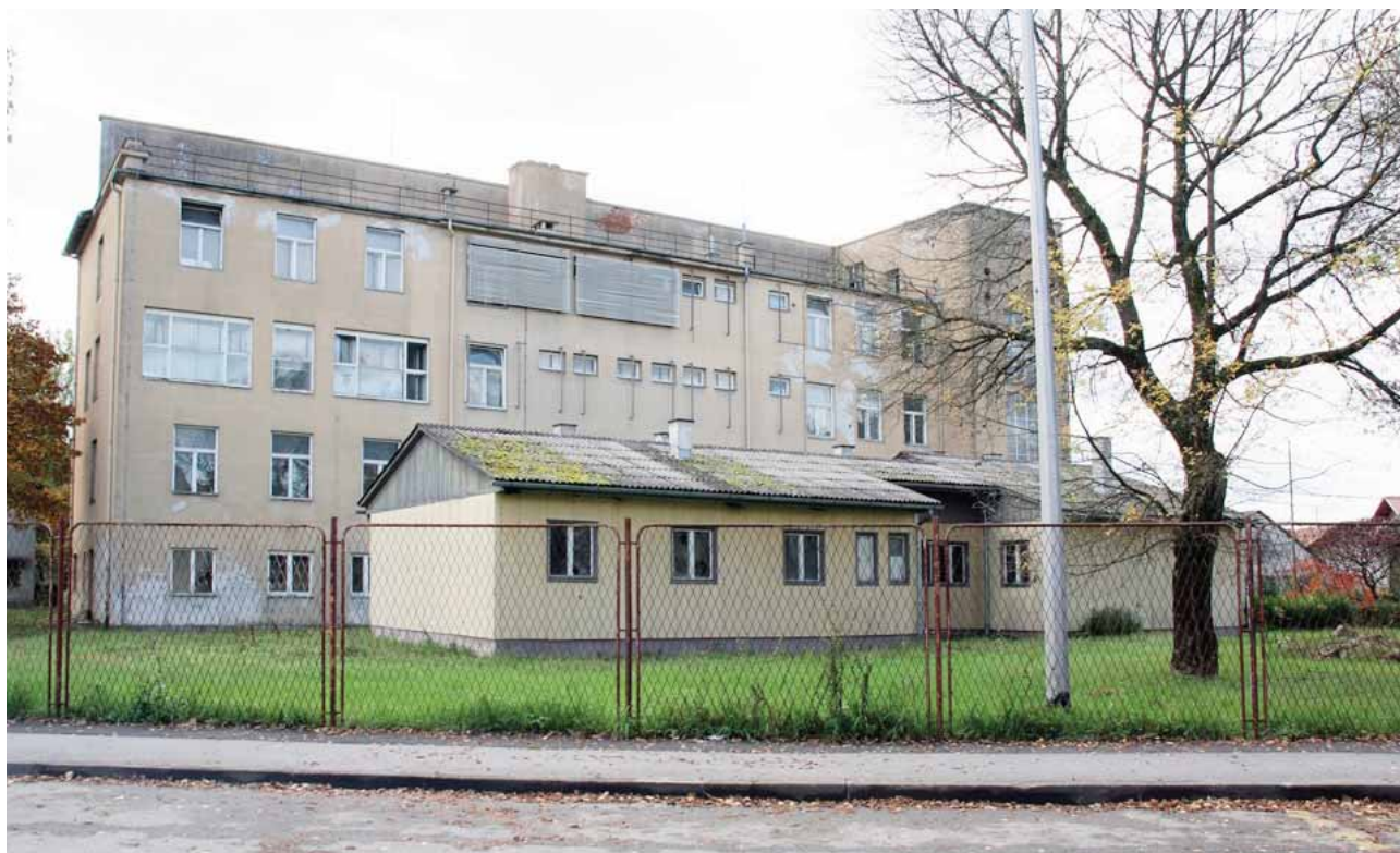
The building in Glina, Croatia, to be reconstructed to accommodate 75 elderly and disabled persons
